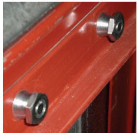
held firmly in position but you should not shear the heads off the nuts, yet.
