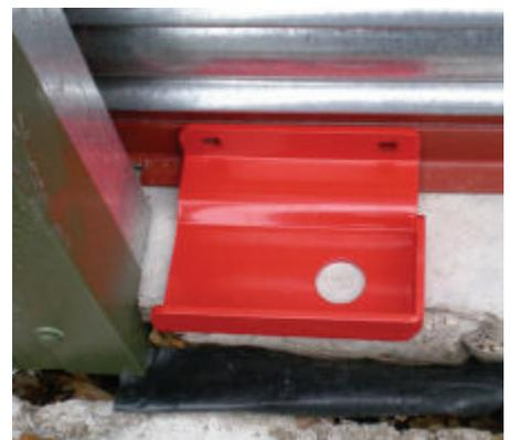
**3. Note:** The recommended gap between the left edge of the plate and the door frame is 20mm.
