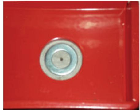
5. Then use the 40mm diameter **Core Drill** to drill to 40mm depth. This will leave a round plug of concrete still in position that needs to be knocked out. That is easier if you now use the **18mm SDS+ drill** bit to drill to 200mm depth, using the pilot hole drilled initially as a guide. Take care to keep vertical as any alignment error will cause the socket to be out-of-line, later.
